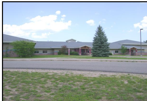
Cherry Creek Elementary School
